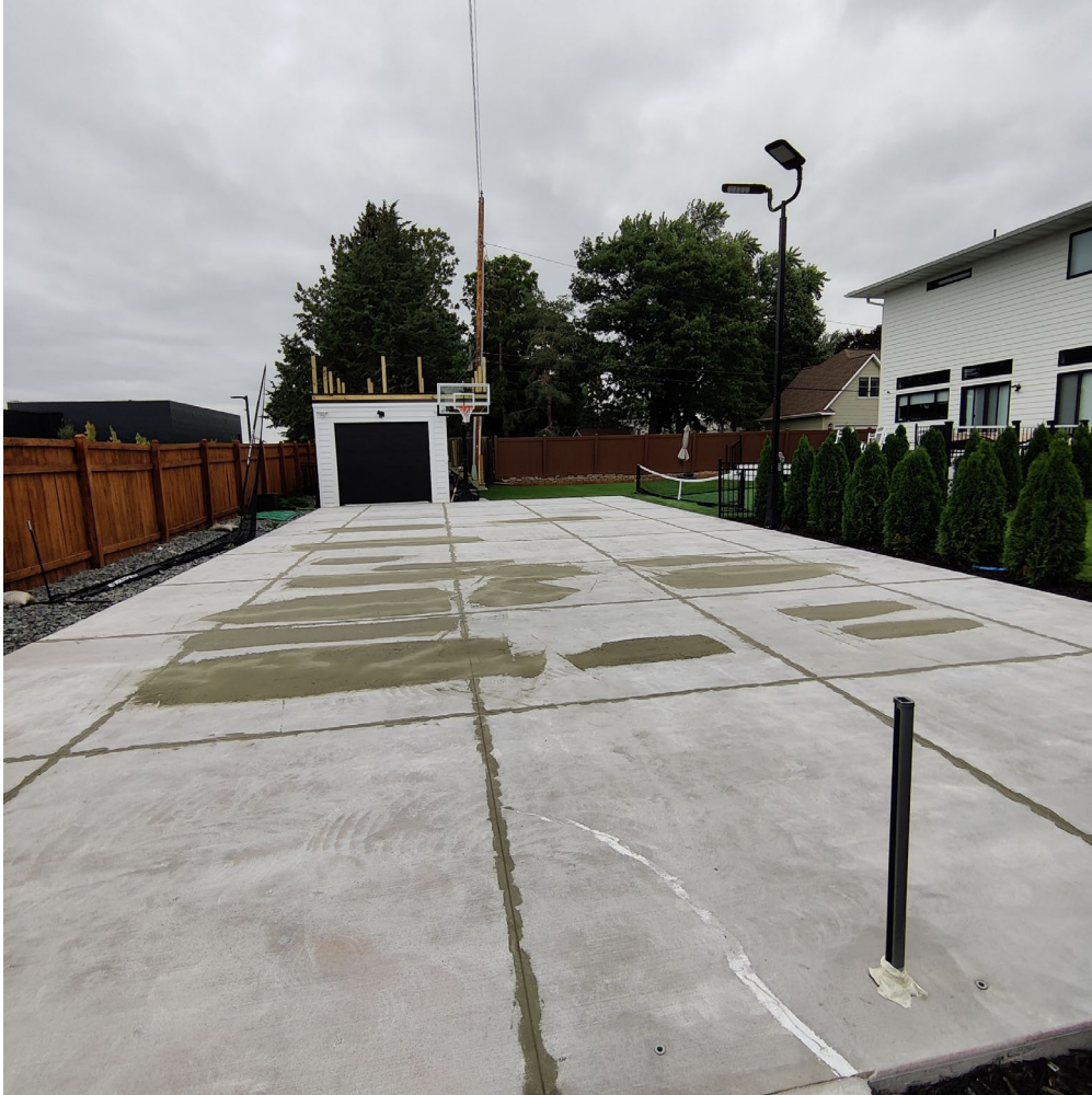
1. Clean Court Surface, Repair Cracks if Applicable
