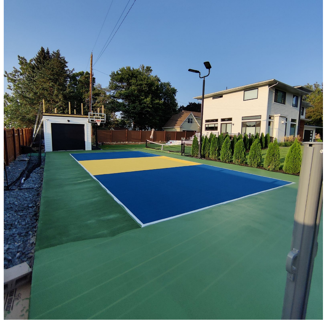
4. Color Coat Perimeter (2 coats)
