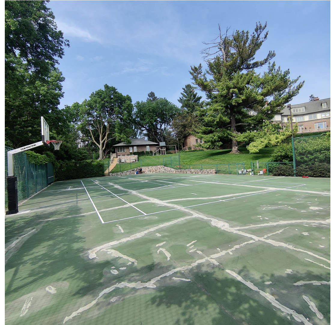
Crack Filling
