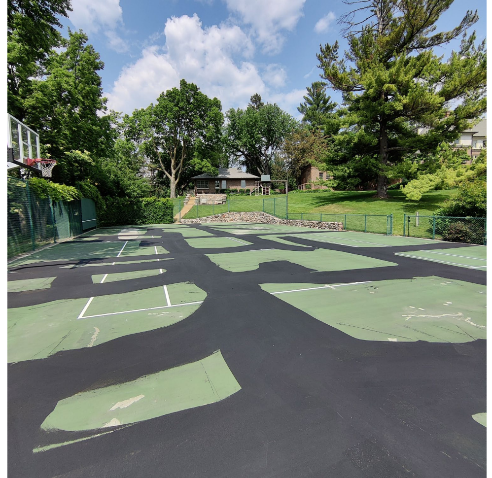
Coat with Acrylic Resurfacer
